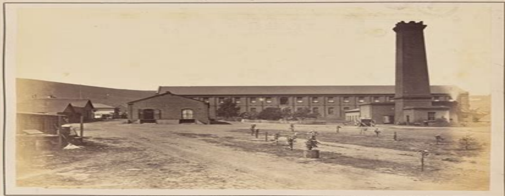
VIEW OF THE CORDAGE FACTORY OF TUBBS & CO., AT THE POTrero, SAN FRANCISCO.
